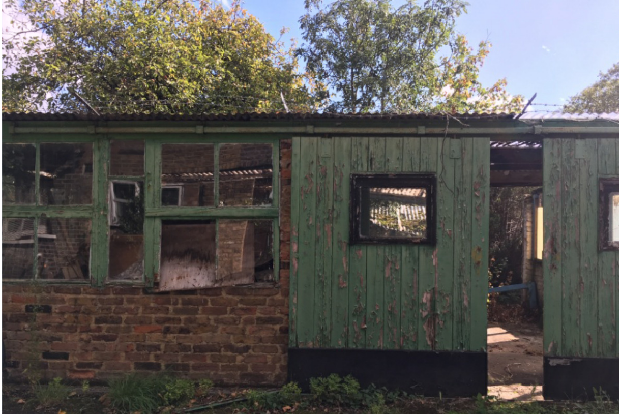
View of one of existing structures on site
