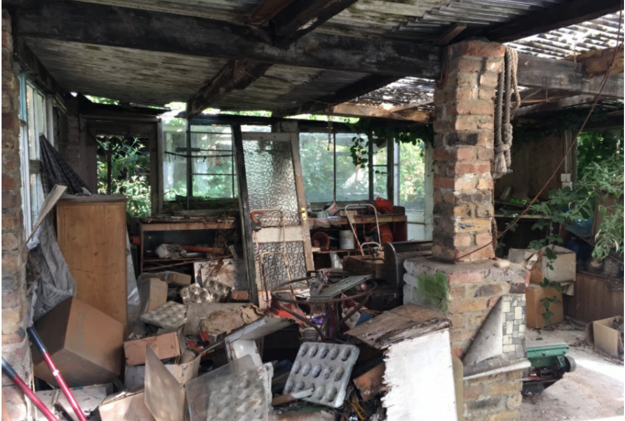
Internal view of one of existing structures on site
